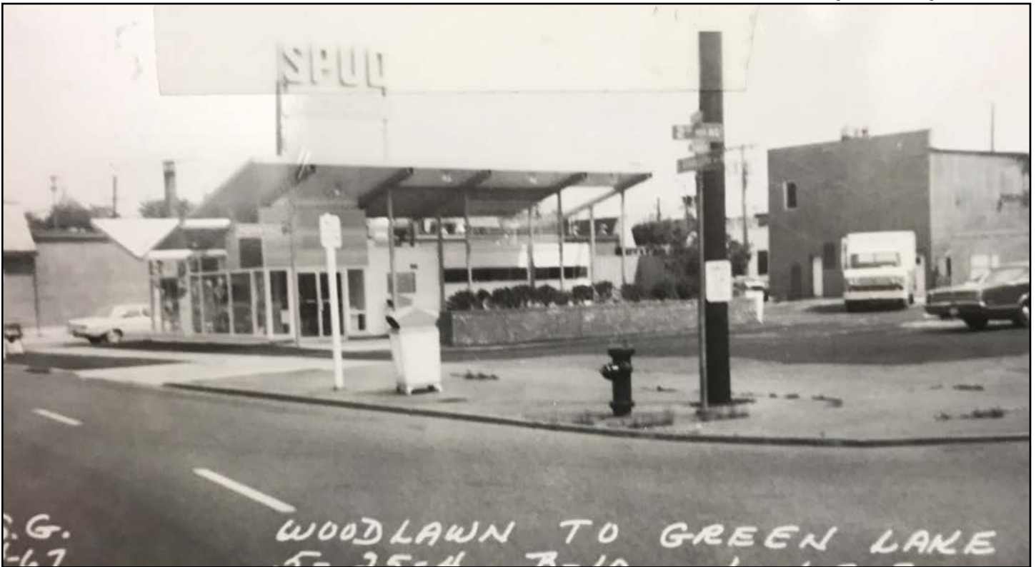
Figure 37 • Spud Fish & Chips in new location with added roof, 1967
