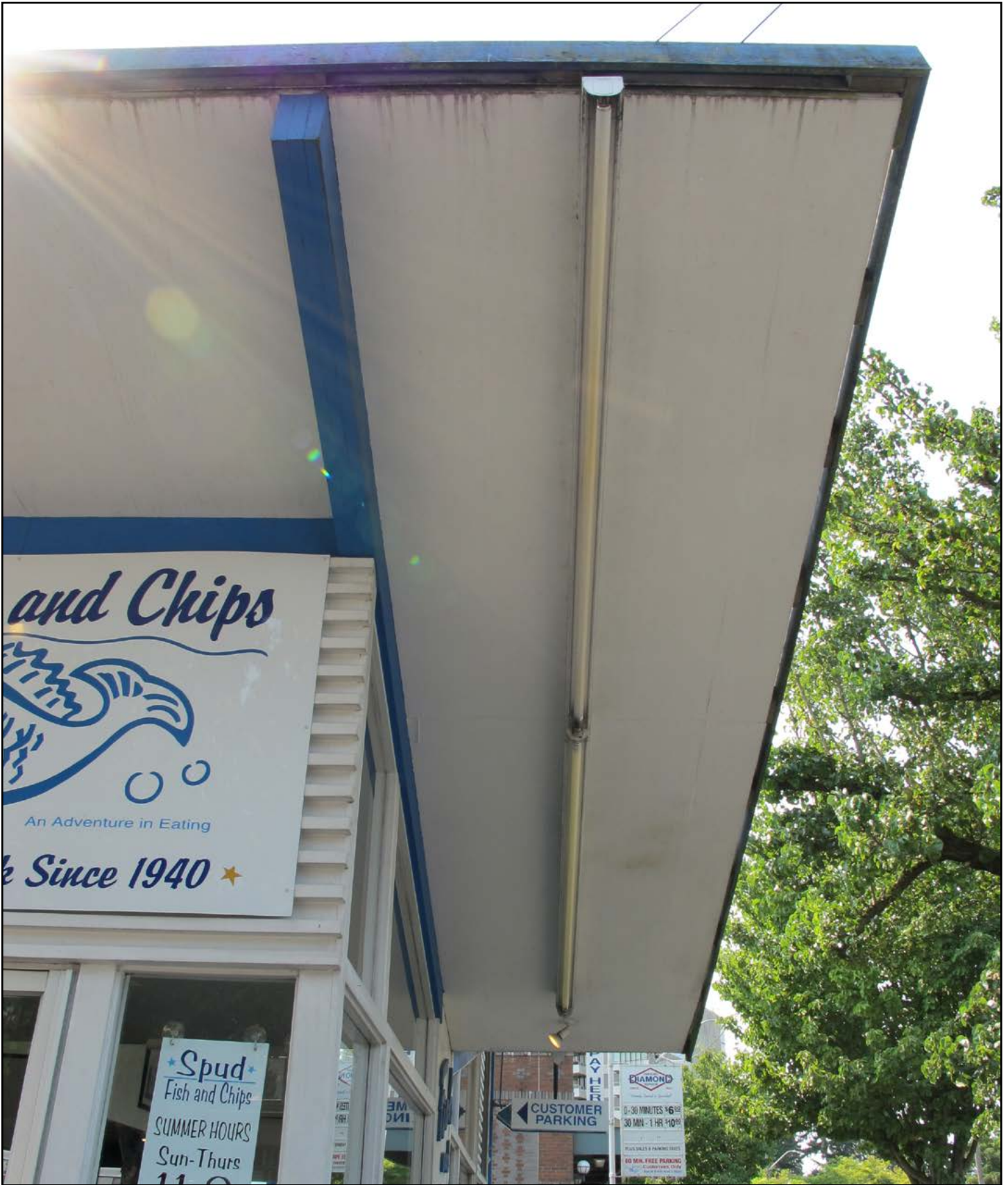
Figure 12 • Spud Fish & Chips Green Lake, detail under northern façade overhang
