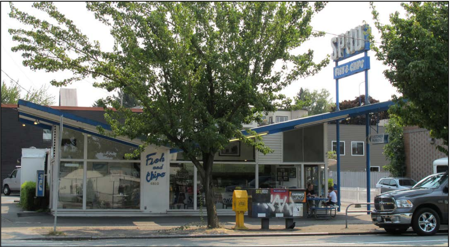
Figure 8 • Spud Fish & Chips Green Lake, northern façade
