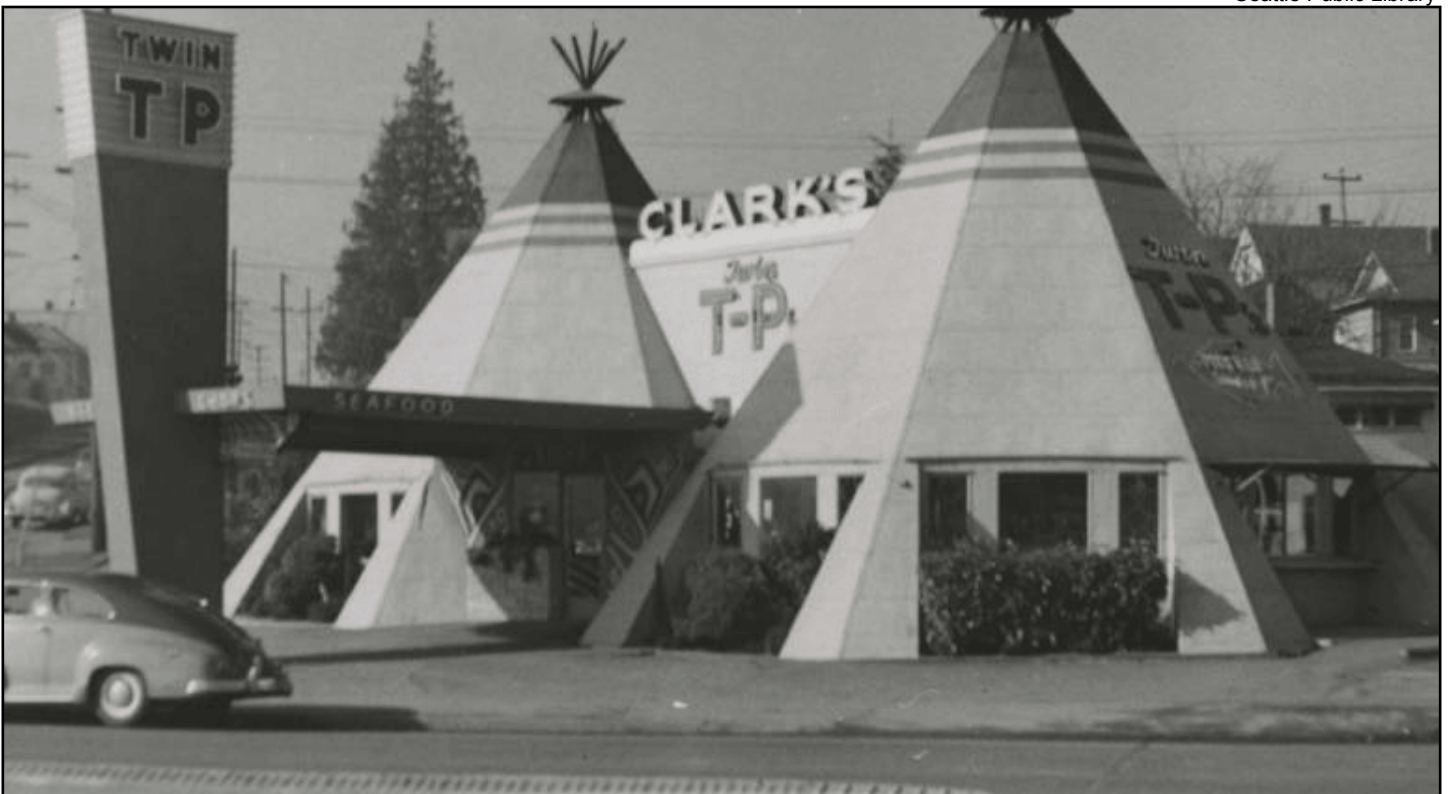
Figure 39 • Twin T-P's (later Twin Teepees, 1937, Delland Harris), 1954
