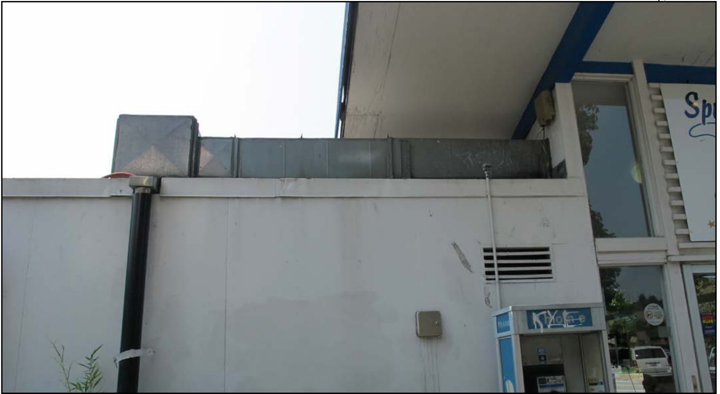
Figure 22 • Spud Fish & Chips Green Lake, eastern façade, detail of mechanical equipment on low-slope roof
