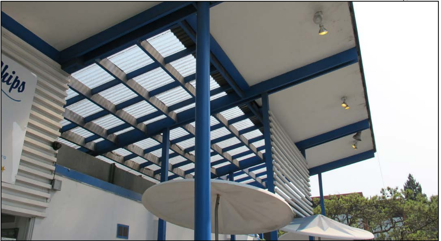
Figure 16 • Spud Fish & Chips Green Lake, western façade, overhang skylights and utility lights
