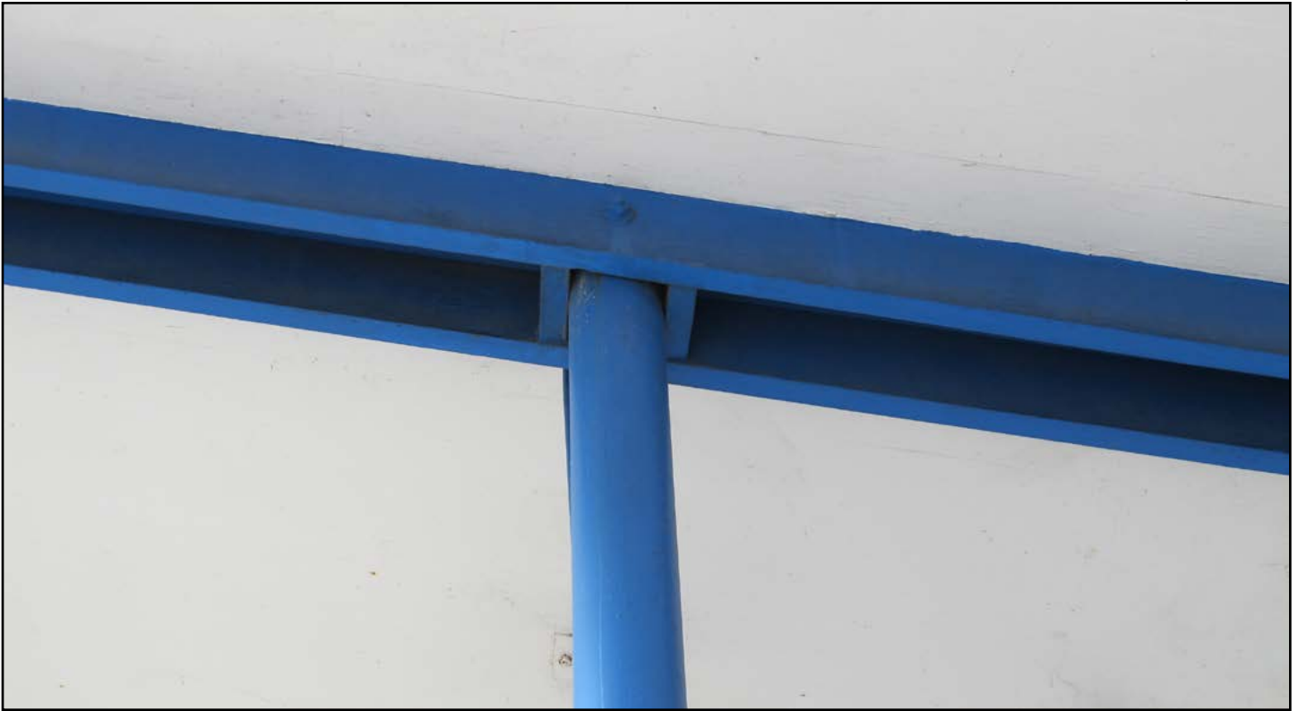
Figure 14 • Spud Fish & Chips Green Lake, western façade, steel column detail
