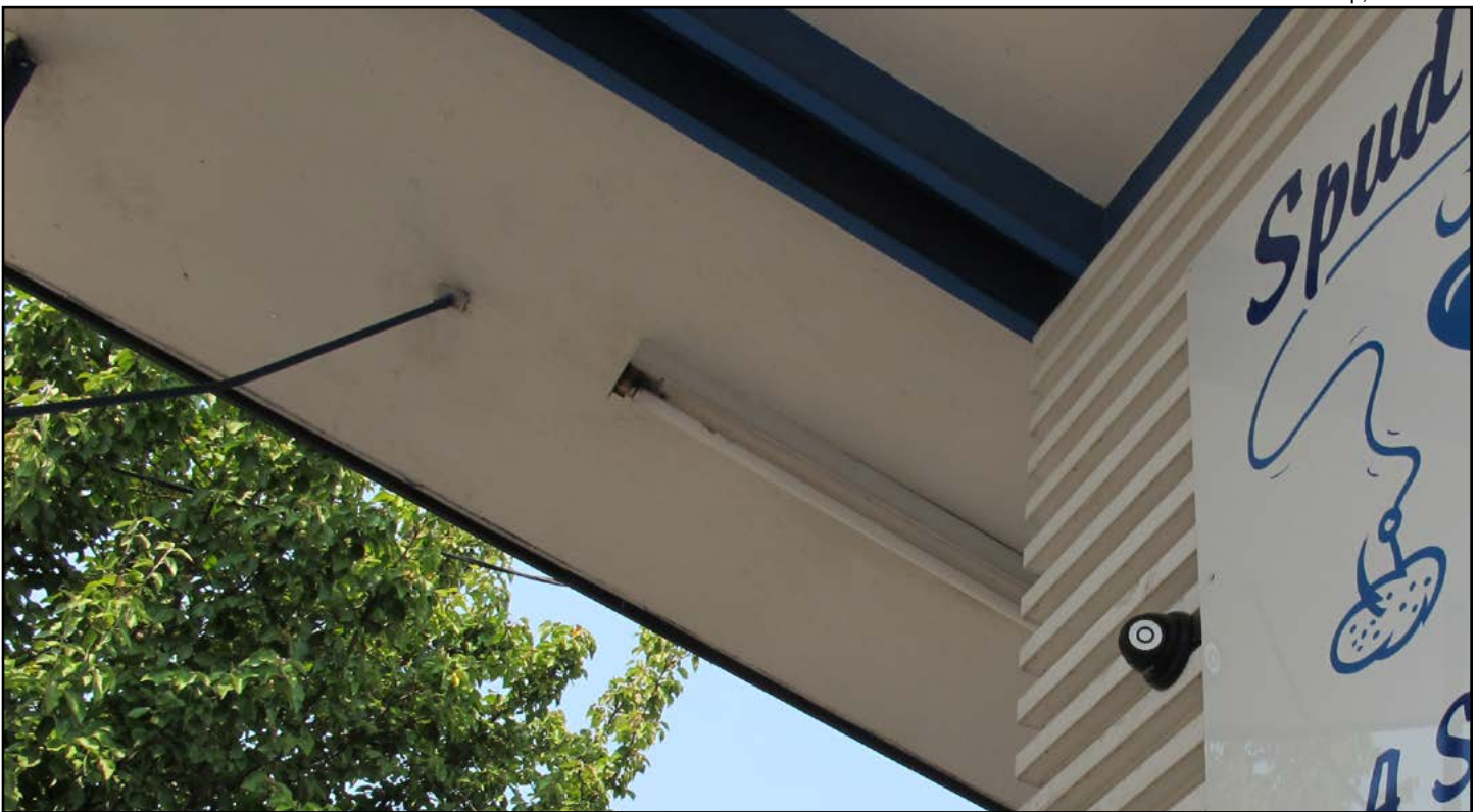
Figure 15 • Spud Fish & Chips Green Lake, western façade, detail of horizontal slats and roof overhang
